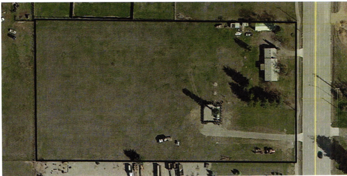
Figure 3: Existing Site Conditions
